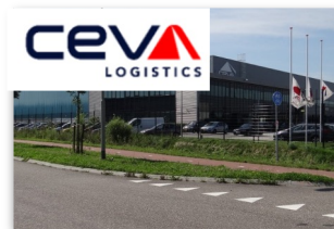
Lightyear Warehouse Consolidation Center (Oostrum, NL)
